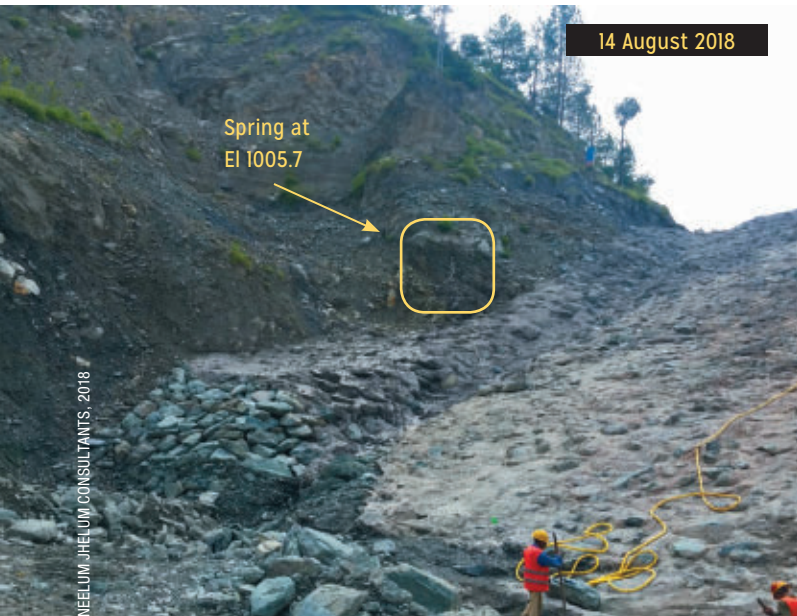
Figure 3: Spring on Downstream Right Bank (left) and Close-up (right).
