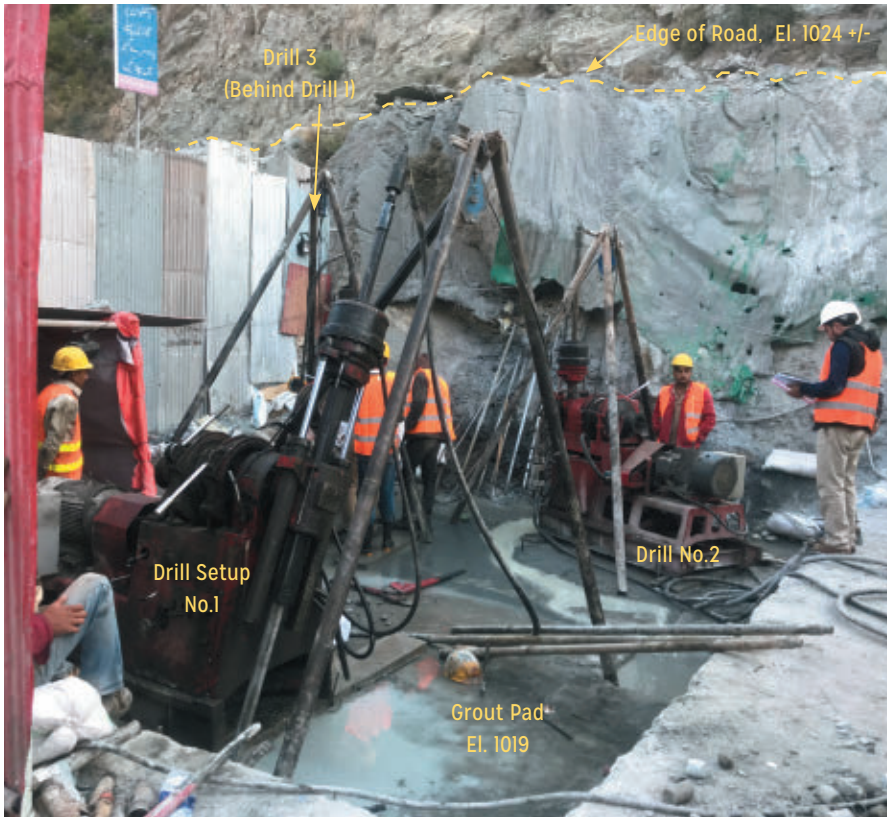
Figure 6: Grout pad at El. 1019 offered approx. 7m x 7m work area.
