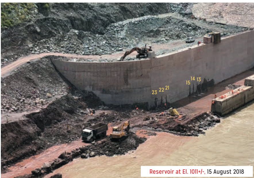
Figure 4: Seepage from Debris Channel Wall Drains.
