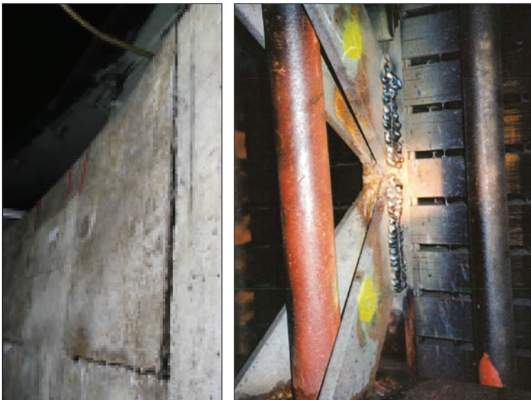
(g) Sole plate grout block protruding from concrete wall towards the shaft.
