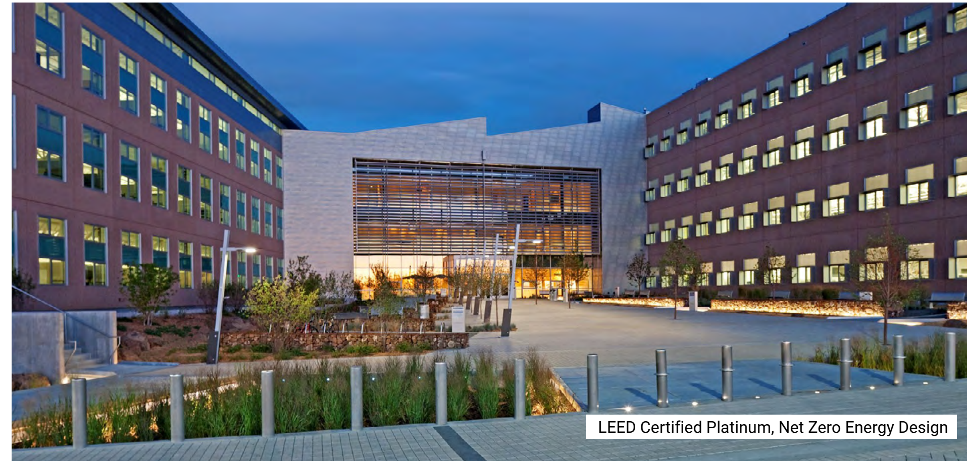
📍 NREL Research support Facility 1 / Golden, CO
